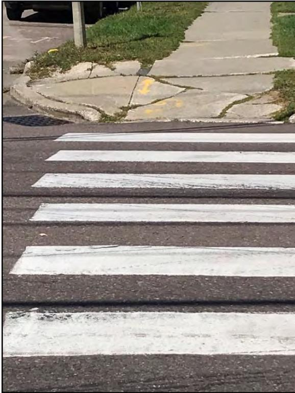
**Photo 6-2: Numerous deficient sidewalk access ramps**
