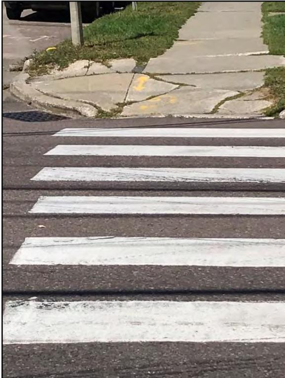
**Photo 6-2: Numerous deficient sidewalk access ramps**
