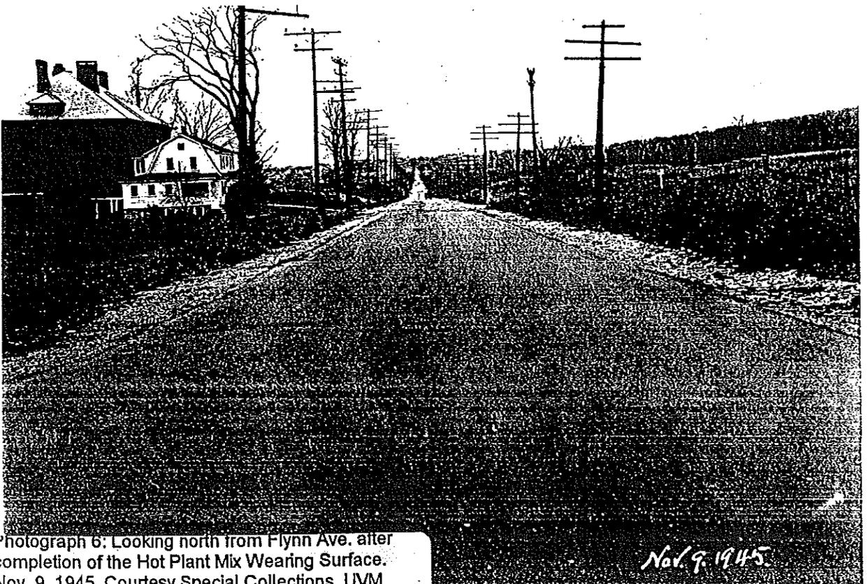
Photograph 6: Looking north from Flynn Ave. after completion of the Hot Plant Mix Wearing Surface. Nov. 9, 1945 Courtesy Special Collections, UVM
